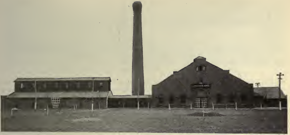
GENERAL VIEW OF THE CAMDEN, N. J., WATER-WORKS
